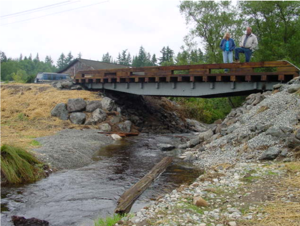
New Railcar Bridge for road crossing Chimacum Creek
