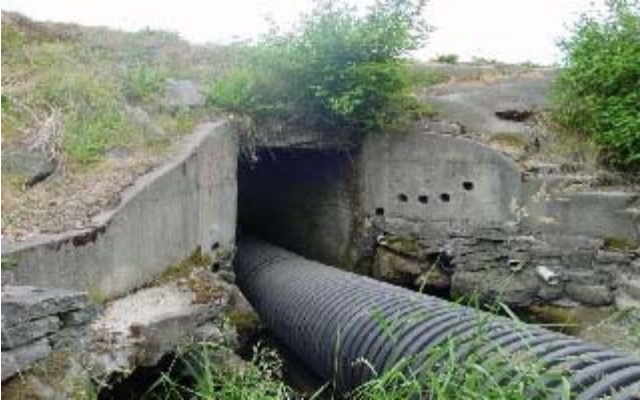
Original Culvert on West Fork of Chimacum Creek
